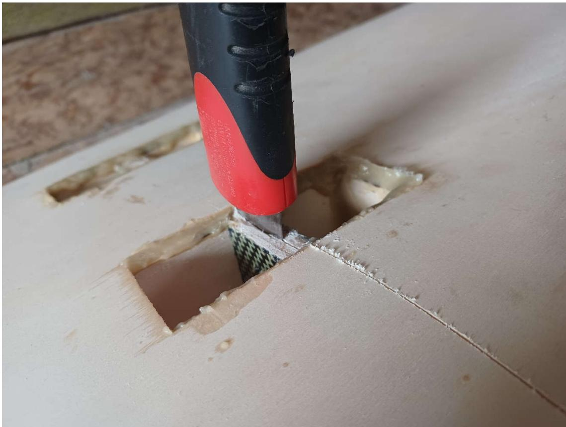
After doing this, you can finally dress the outside faces of the bulkheads with the mesh. Re-drill the connecting holes after the epoxy has set on the mesh, epoxy also the inside edges of the holes, or use small copper or stainless tubes of the same diameter as the screws to protect the ply from being abraded by the screws.
