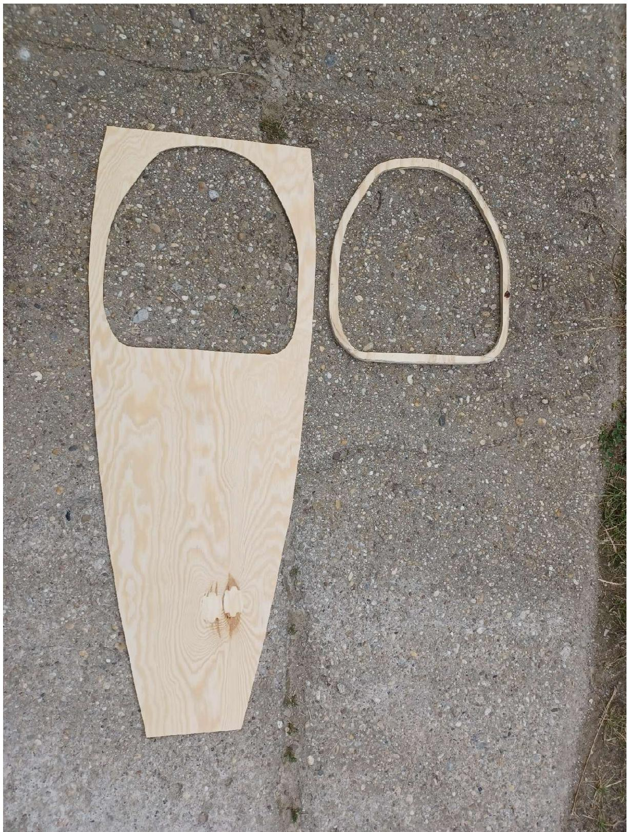
24. Cut the cockpit coaming from the 9mm plywood. Use the plywood leftover piece that resulted from cutting the cockpit hole as a template
